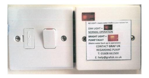
Within the mechanical service cupboard in your property alongside the switch which controls the power to the submersible pump inside your rainwater harvesting tank, there is a warning light. The status of this light is clearly described an illustrated on the above picture and as follows:
